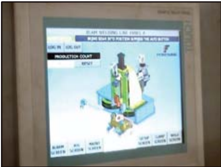
Large display of system status
